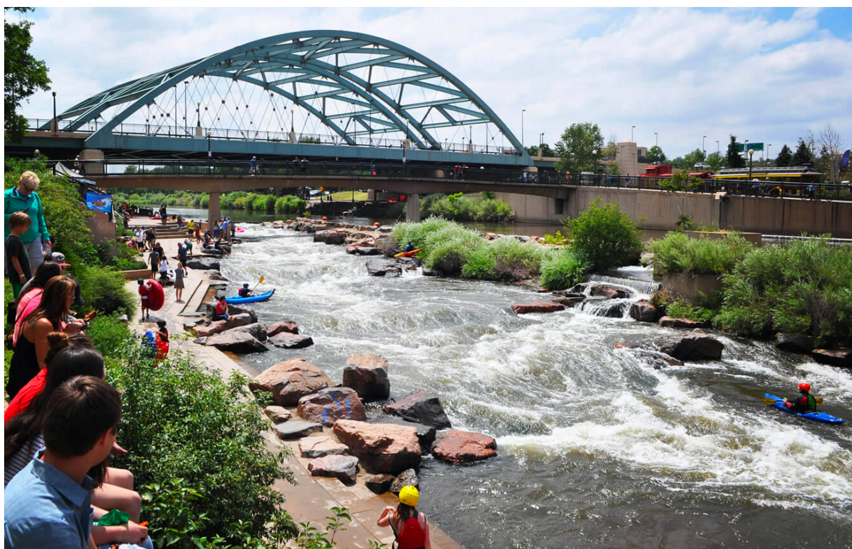
Figure 2-13. Confluence Park on South Platte River in Denver, CO receives accolades as a “top 10” destination in the city for its water-based recreation and connectivity to trails, restaurants, shops, and services. The grouted rock construction of five Class III whitewater features also serve to dissipate an eight-foot hydraulic drop over a 400-foot river reach. Constructed in 1995, the park has served visitors for over thirty years “without serious injury” or “significant bed degradation” and “virtually no maintenance cost (Merrick, 2019).” As infrastructure ages, transformations of channels and drop structures in Walnut Creek’s watershed become opportunities to support multiple ecosystem services within engineered channel infrastructure through urban areas. Services of creeks can include play and communal celebration of creek corridors as public aquatic parks while also allowing fish passage and promoting flood safety. Precedents for multi-functional planning of urban river corridors, such as the greenways being integrated with development along Denver’s South Platte River, deserve further consideration (Appendix E).
